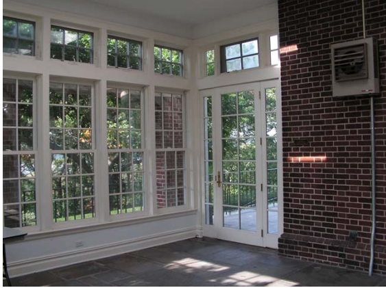
Sun Porch, Northwest corner
