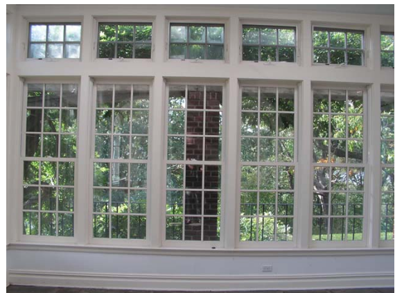
Sun Porch, West Wall
