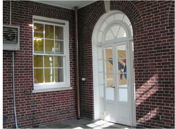
Sun Porch, Northeast corner, with door to Sunroom
